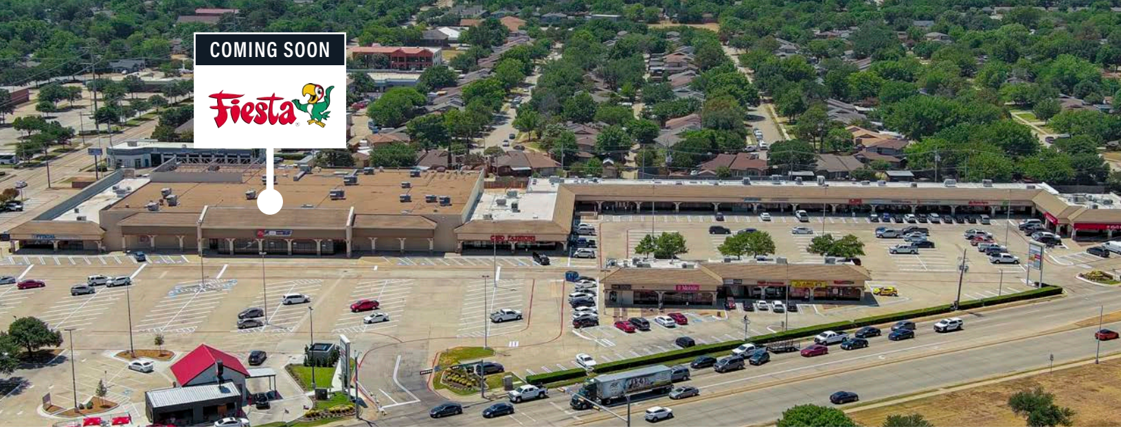
At Valley Square in Lewisville, grocer Fiesta Mart plans to open in a former 24 Hour Fitness anchor space.
