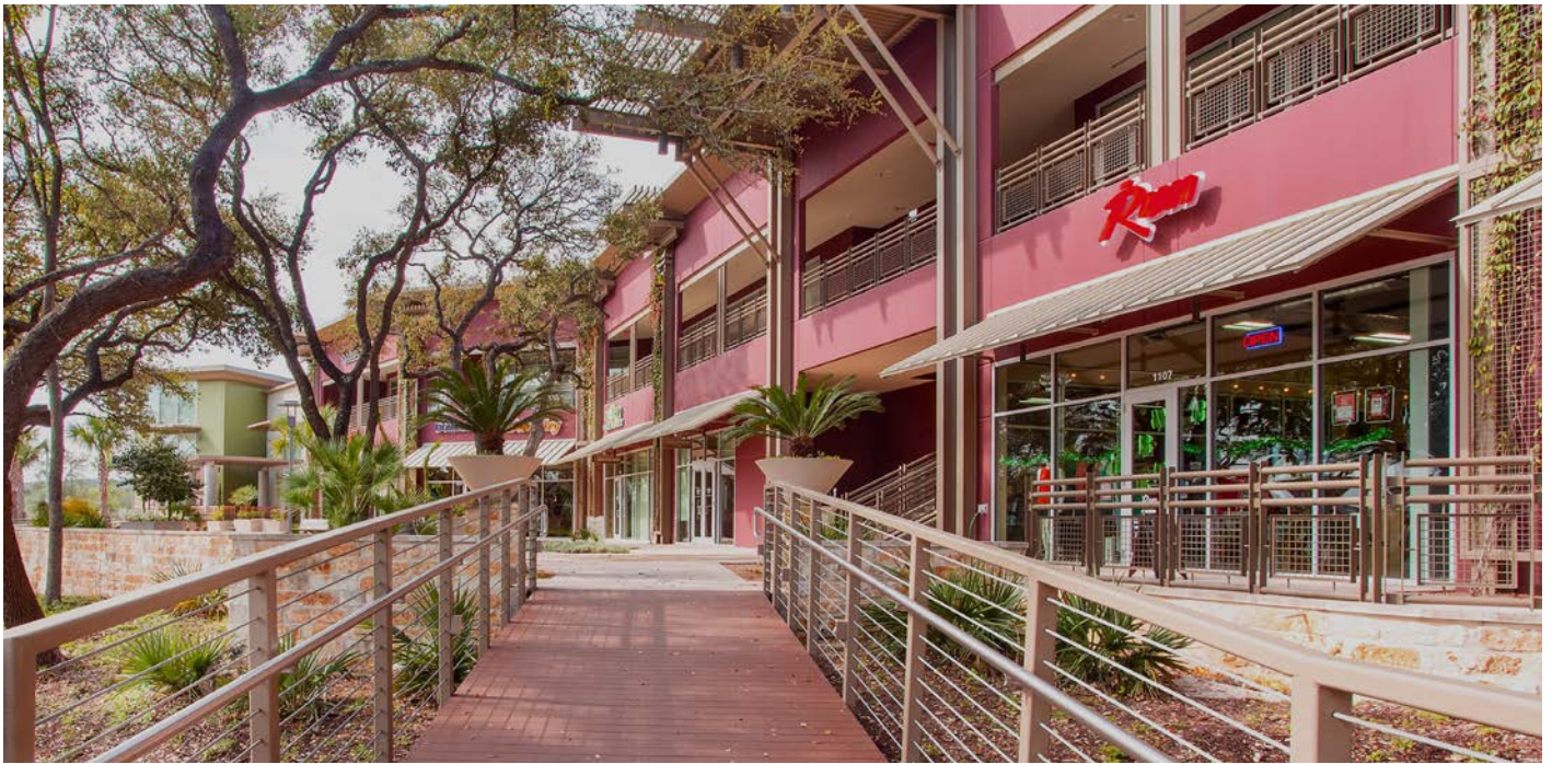
The fully leased Dominion Ridge project is a prime example of the high occupancy rates to be found at centers throughout the market.
